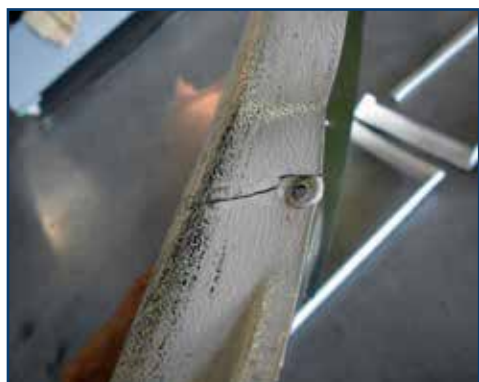
Typical condition of a 40-year-old plastic window frame.
