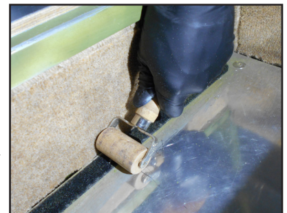
Firmly pressing velcro in place with a wood roller.
