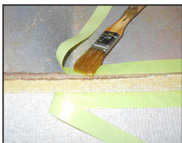
Neatly applying adhesive to the rough backing surface of carpet.
